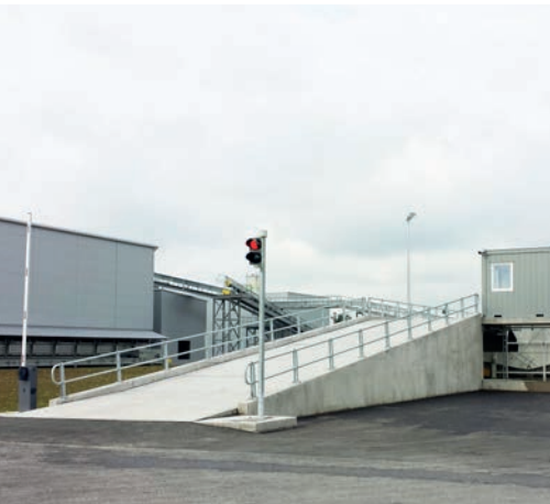
Intake with walking floor, 25 t/h
