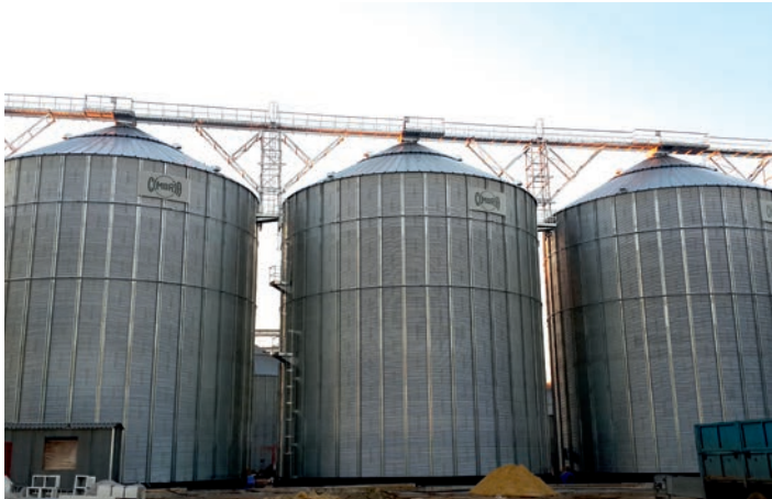
Ecoprod site under construction
