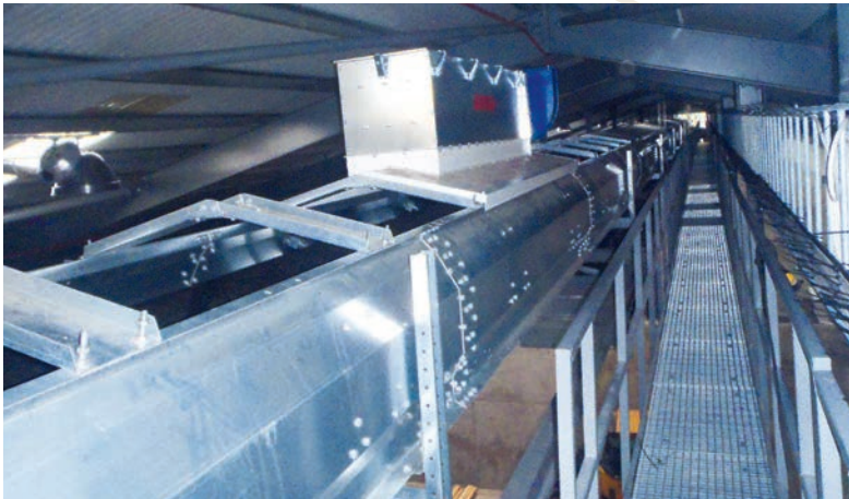
Longitudinal belt conveyor 300 TPH with spot filter
