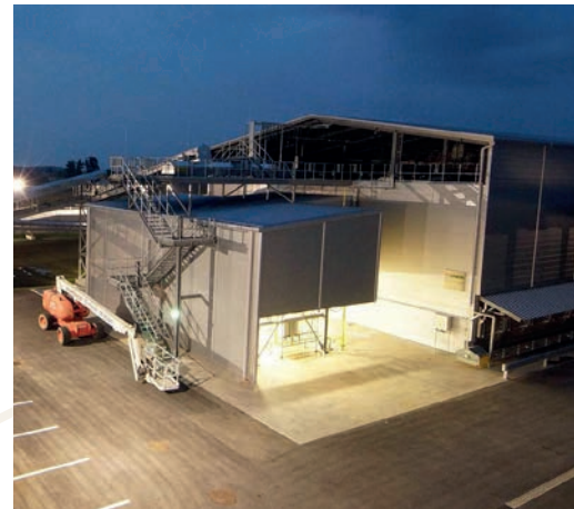
Ear corn dryer, filling capacity 1,200 t
