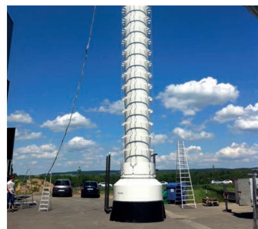
Test of V1200 loading chute in Litomysl
