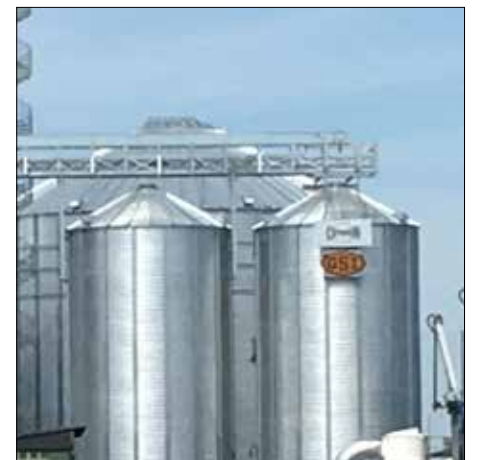
The system in Hammenhög consists of an intake system with pre-cleaning and silos for storage of wet grain before drying, an ECO-Logic™ dryer, storage silos and connection to existing flatbed storage
