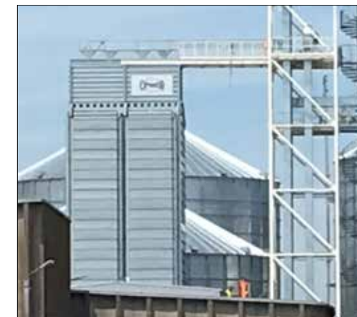
The system in Hammenhög consists of an intake system with pre-cleaning and silos for storage of wet grain before drying, an ECO-Logic™ dryer, storage silos and connection to existing flatbed storage
