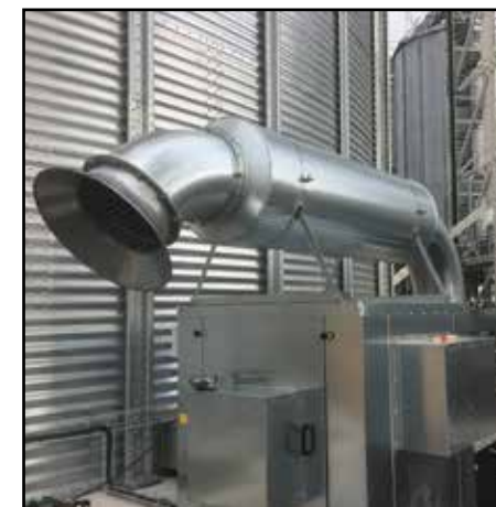
The ECO-Logic™ is provided with centrifugal fans with limited noise emission
