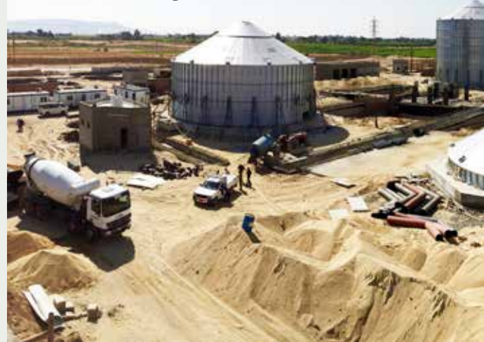
Installation work in progress
