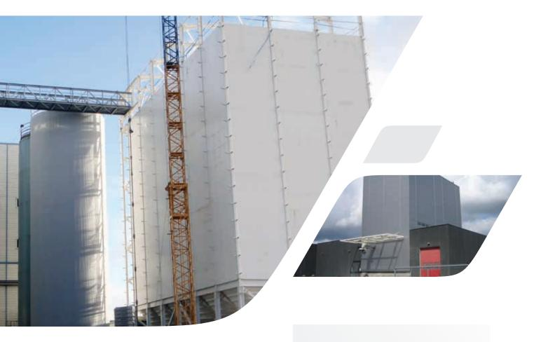
Cimbria square silos are manufactured to store many different smaller quantities of grain products, with capacities of up to 20,000 m<sup>3</sup> or even higher. Built with heavy, trapezoidal, or face-plated steel plate, and with cell sizes up to 4m x 4m, they can be delivered in several combinations. Each silo is individually and precisely designed to meet the customer's specific demands.
