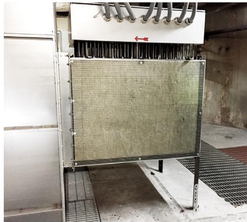
Felleskjøpet: Electric calorifier with an output of 770 kW
